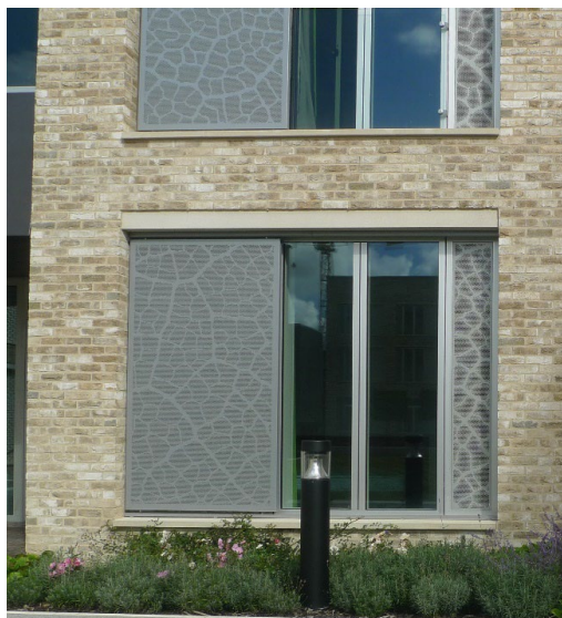
Figure 6. Image of acoustically attenuated openings: North West Cambridge student residences (images courtesy of Nick Conlan, Apex Acoustics).
